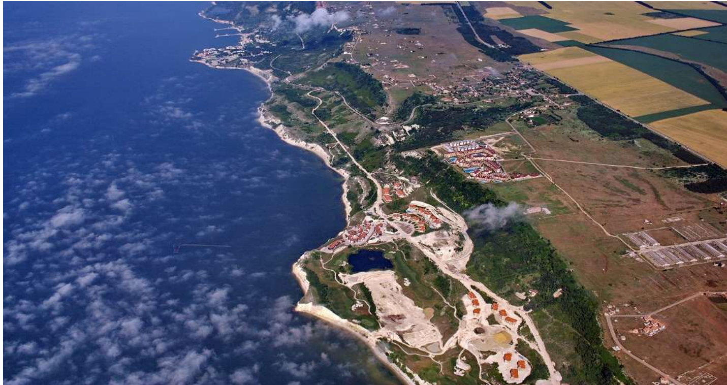
Kavarna Municipality. Patchwork, uncontrolled completion
