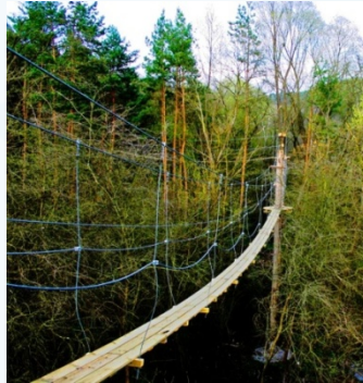
Fig.: Cableway, ipolytarnóc (HU)
