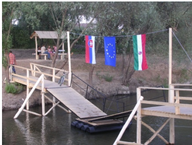
Fig.: Footbridge between village Ipeľské Predmostie (SK) and Drégelypalánk (HU)
